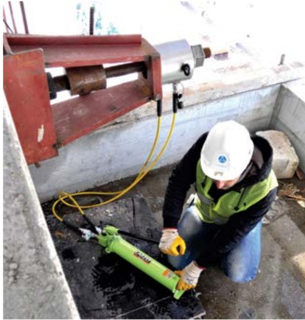
The system was put into practice in cooperation with Strainstall UK, POLARKON's solution partner in Turkey, and also consultancy of METU Department of Civil Engineering. Data collection system installed on site measures the axial tension loads on each rod, recorded every hour, and the information sent to the main service provider.
